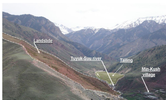
Fig. 3 The common view of the tailing and landslide in valley of river Tuyuk-Suu.
