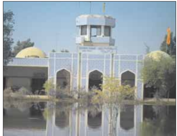
Fig 4. Sehwan: Airport under water
