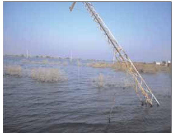
Fig 10. Khairpur Nathan Shah-Dadu: Damage to Installations
