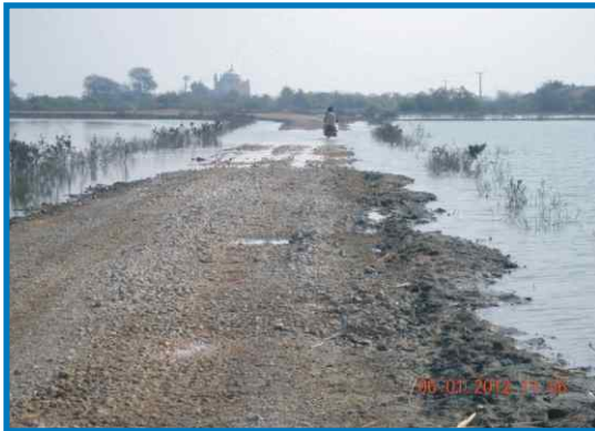
Damage to Infrastructure
