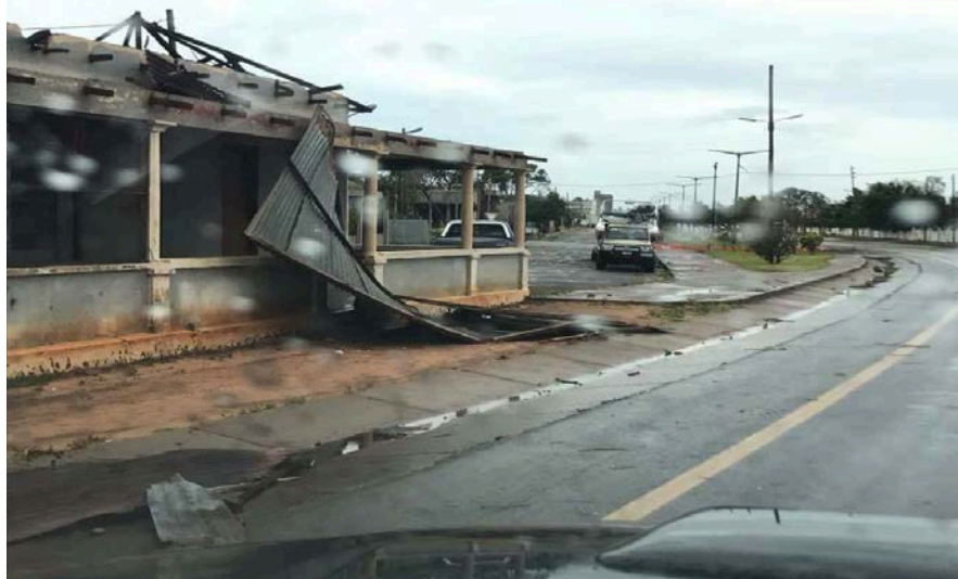
House destroyed at Maxixe City
