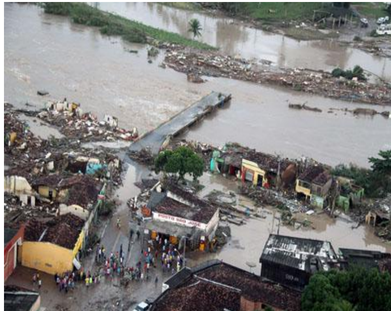
Bridge flooded and destroyed
