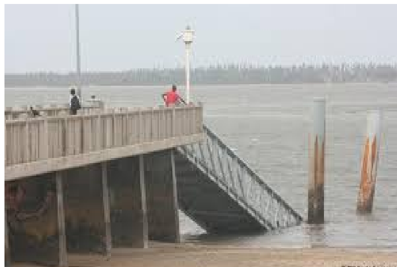
Bridge destroyed (Maxixe-Inhambane crossing)
