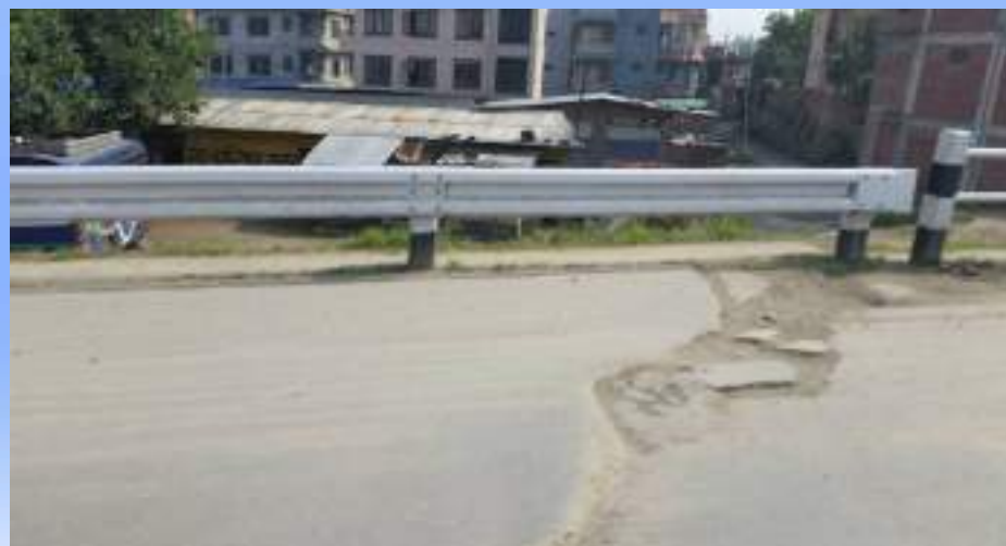
Uneven settlement of junction of cross-river bridge ( right )
