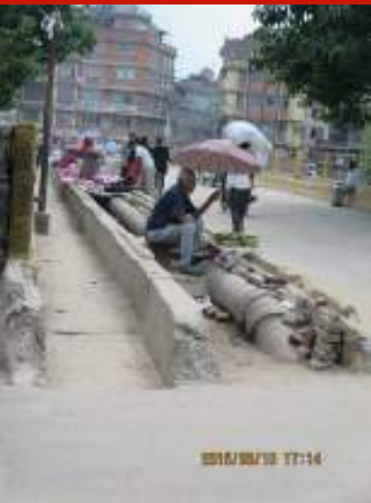
Feed mains (Cast iron pipe)
