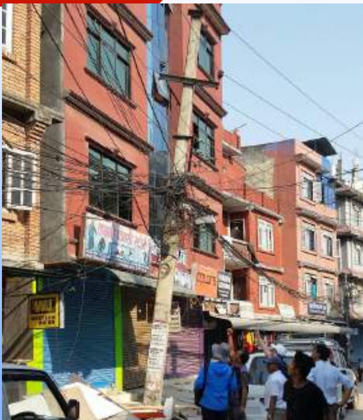
Urban electricity supply & communication line ( top )
