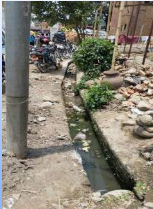
Open drain (confluence of rainwater & sewage)
