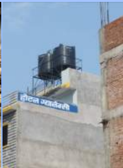
Water storage tank
