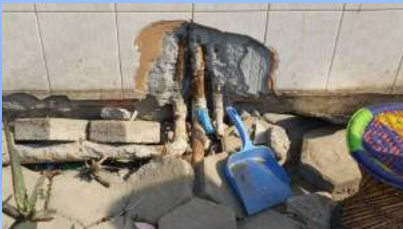
Inlet branch pipe (Galvanized pipe)
