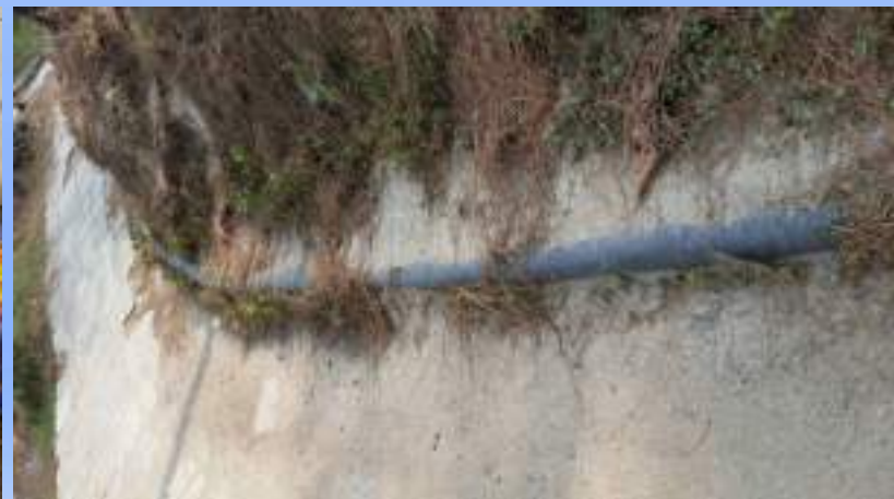
Range pipe (Exposed installation , PE pipe)
