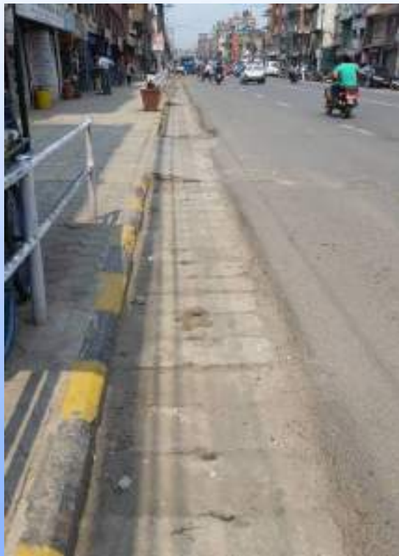
Drain cover plate (confluence of rainwater & sewage)
