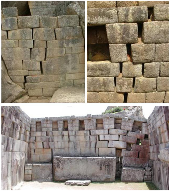
Fig. 3 Examples of cracks collected in the archaeological structures and buildings (photos by D. Spizzichino)
