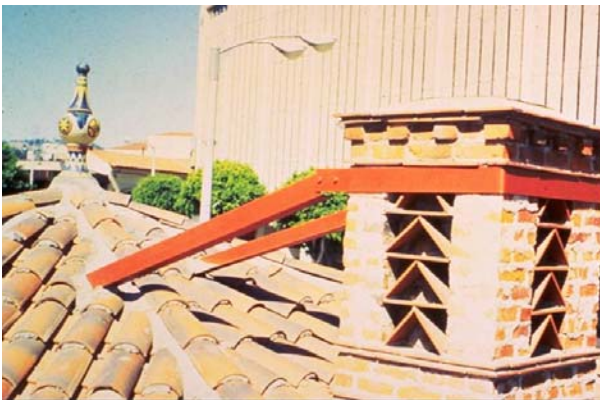
Figure 6-5: Typical Chimney Bracing
