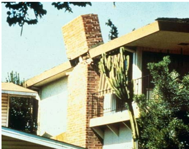
Figure 6-4: Typical Chimney Damage
