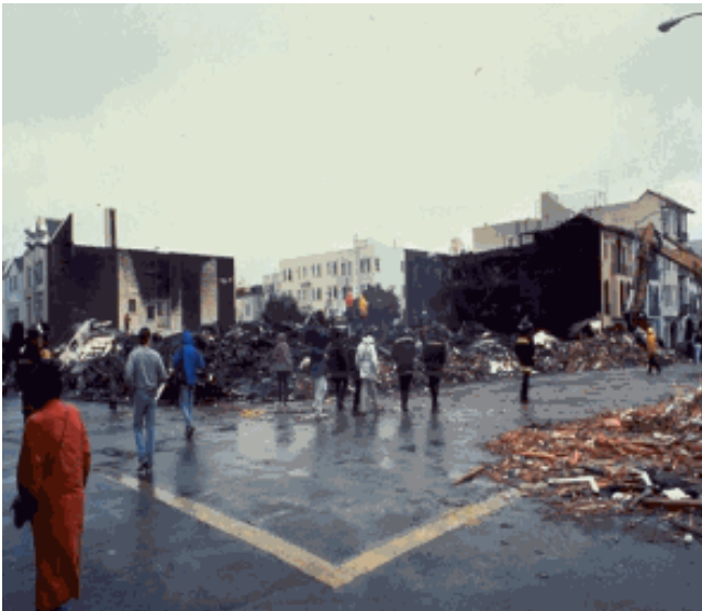
Figure F-10: Typical Damage to URM Buildings due to Poor Walls, Connections
