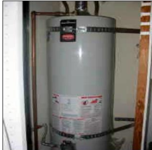
Figure 6-17: Typical Bracing of Hot Water Heater
