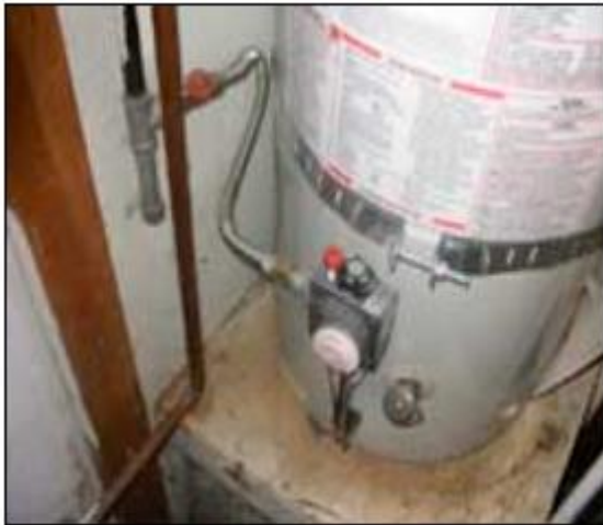
Figure 6-20: Typical Flexible Connection
