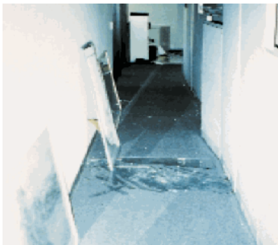
Figure 6-26: Typical Wall Hanging Damage
