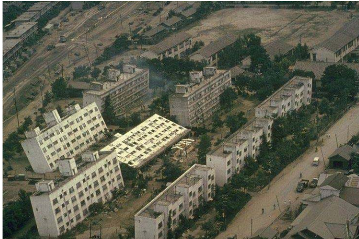
Figure 2-5: Earthquake Damage Due to Liquefaction
