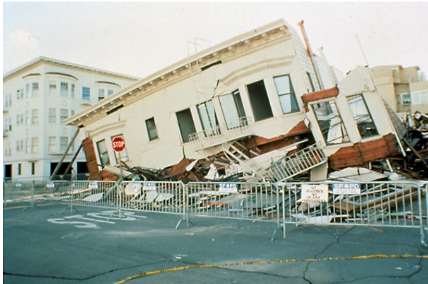
Figure 2-2: Earthquake Damage Due to Ground Motions
