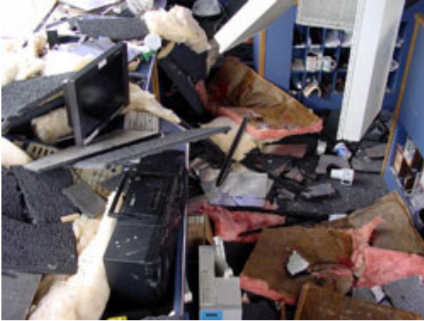
Figure 6-24: Typical Equipment Damage
