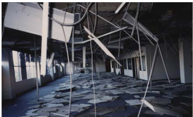
Figure 6-9: Typical Suspended Ceiling and Lighting Fixture Damage
