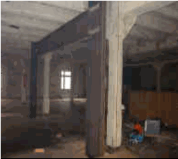
Figure F-12: Typical Moment Resistant Frame
