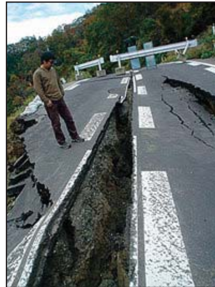
The Niigata Chuetsu earthquake caused large-scale destruction.
