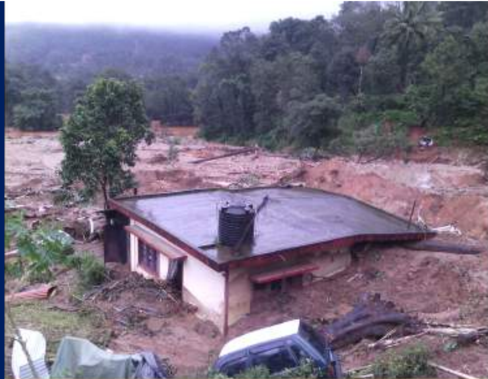
A house destroyed by landslides in Kaloor near Madikeri.
