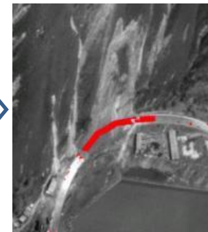
Damaged road segment
