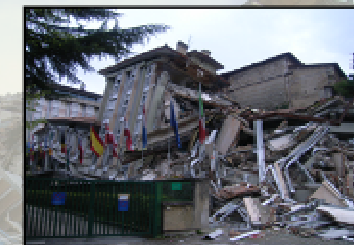
Field photo from L'Aquila earthquake
