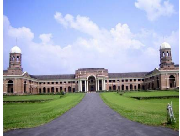
Pic 2. FRI main building
